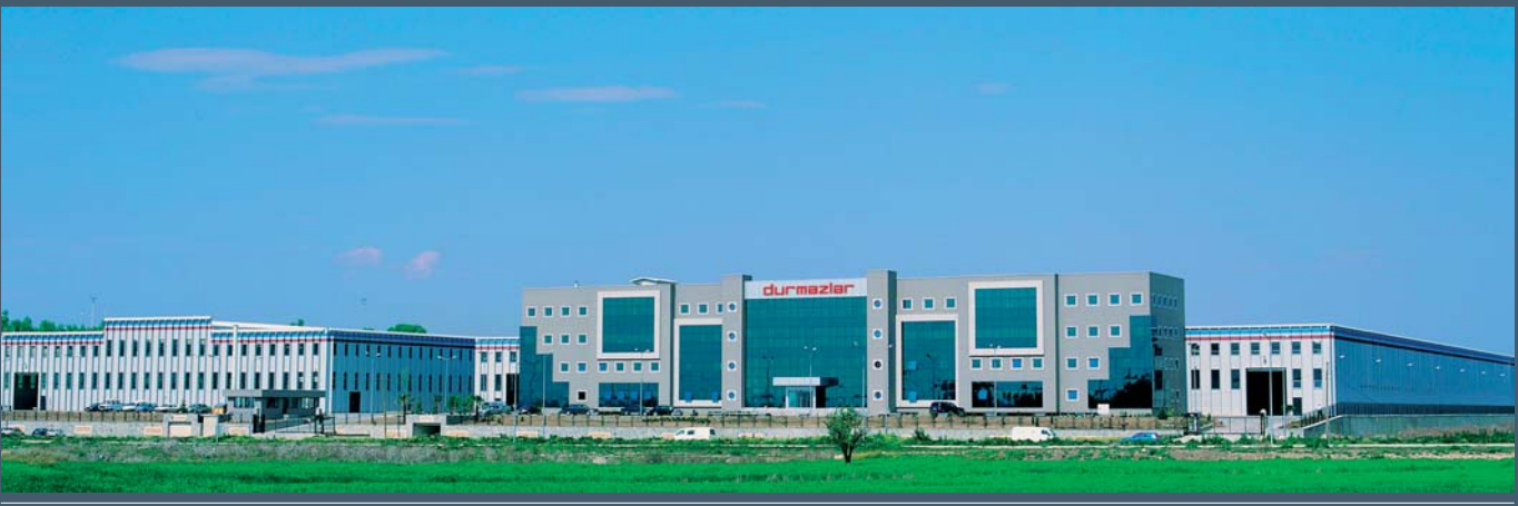
Durmazlar Headquarter & Ataevler Plant
